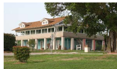
Mound House During Restoration
