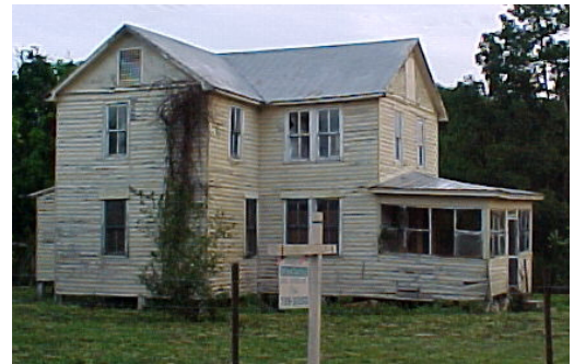
Flint house before restoration
