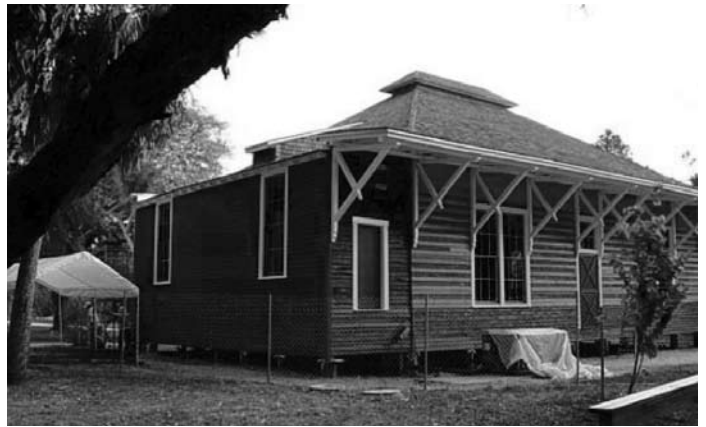
Above: South side of Art Hall Main building Below: North side of Art Hall Main building The roof deck underside, fascia and brackets along with casings received one coat primer and 2 coats white paint. Siding is a mix of original and new.
