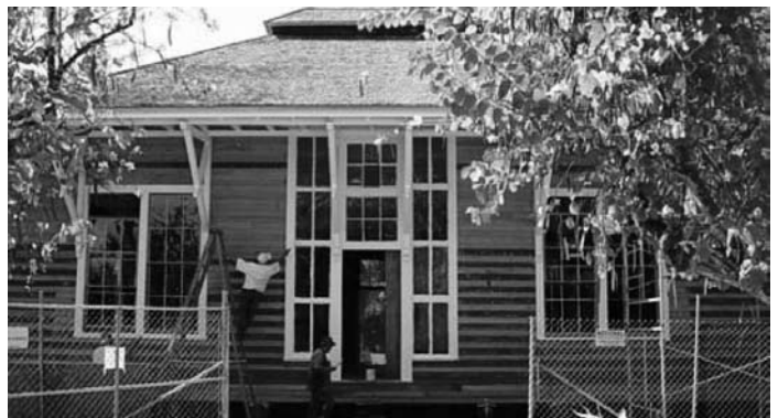
Above: South side of Art Hall Main building Below: North side of Art Hall Main building The roof deck underside, fascia and brackets along with casings received one coat primer and 2 coats white paint. Siding is a mix of original and new.
