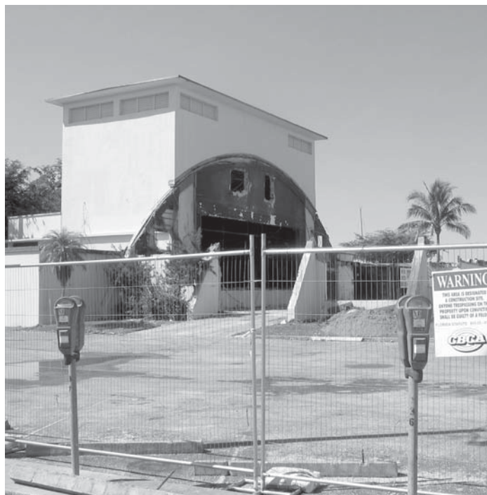
Demolition of the Exhibition Hall
