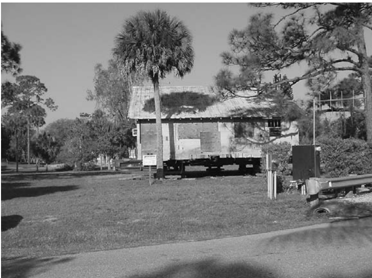
Nutting House: front elevation on Tennessee
