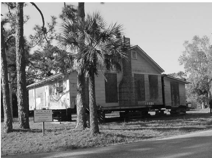
Nutting House: front elevation on Tennessee, side on Pennsylvania
