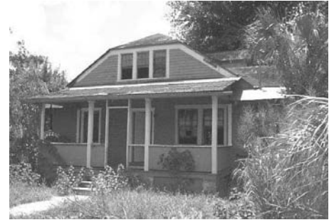
Williams-Packard House: front elevation before move
