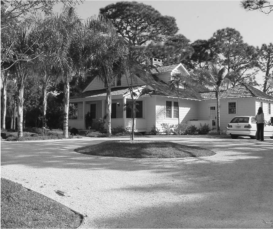
Williams-Packard House Restored: front elevation
